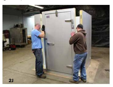
Install right front corner panel making sure panels are flush on top and panel to panel (see figures 2K).
