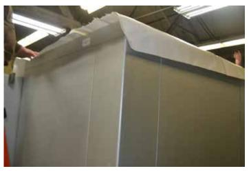
Snap a chalk line approximately 51" from edge of walk-in. Line up tab on membrane roof with chalk line.
