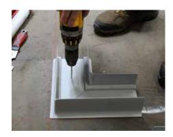
• Slide walls into channel of screed. Lock walls lining up top corners of each wall.
