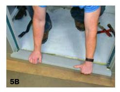
• Attach sill plate to inside top of floor panel with 3 self-tapping screws (see figures 5C).
