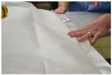
Unroll roof cap membrane to nest tab and fasten. When fastening remaining tabs, check often to make sure all slack in roof cap is pulled taught.
