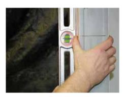
Install door frame and clamp into place.
