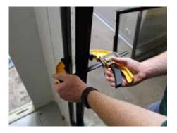
Once the frame is clamped firmly in place and is level, using the screws provided, screw the glass door frame to the buck opening.
