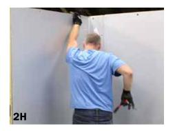
Install left front corner panel making sure panels are flush on top and panel to panel (see figure 2I)
