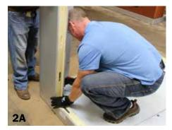
• Back wall panel next to corner panel, lock panels together starting with top lock, then middle lock and bottom lock, making sure panels are flush (see figures 2B, 2C, 2D, & 2E??).
