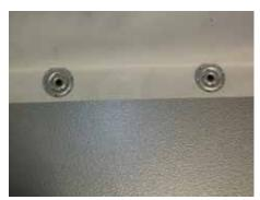
• Fasten reverse tab to building wall using Duro-last plates. Plates will be secured to wall using appropriate screws. Fastened on 6" centers (image).
