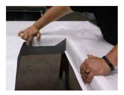
A bead of silicon should be put on the membrane roof prior to dropping unit through the opening. After
