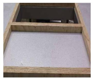
Install membrane roof according to instructions, pulling roofing material over wooden curb.
