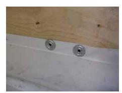
• Install 6" X 6" wall flashing, using appropriate screws, and seal with caulking (image).
